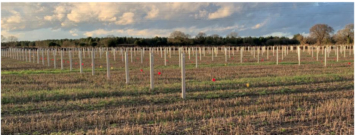
Plate 11-28 Mounting Structure Piles being Installed (taken at Tiln Farm, Retford, in January 2023)
