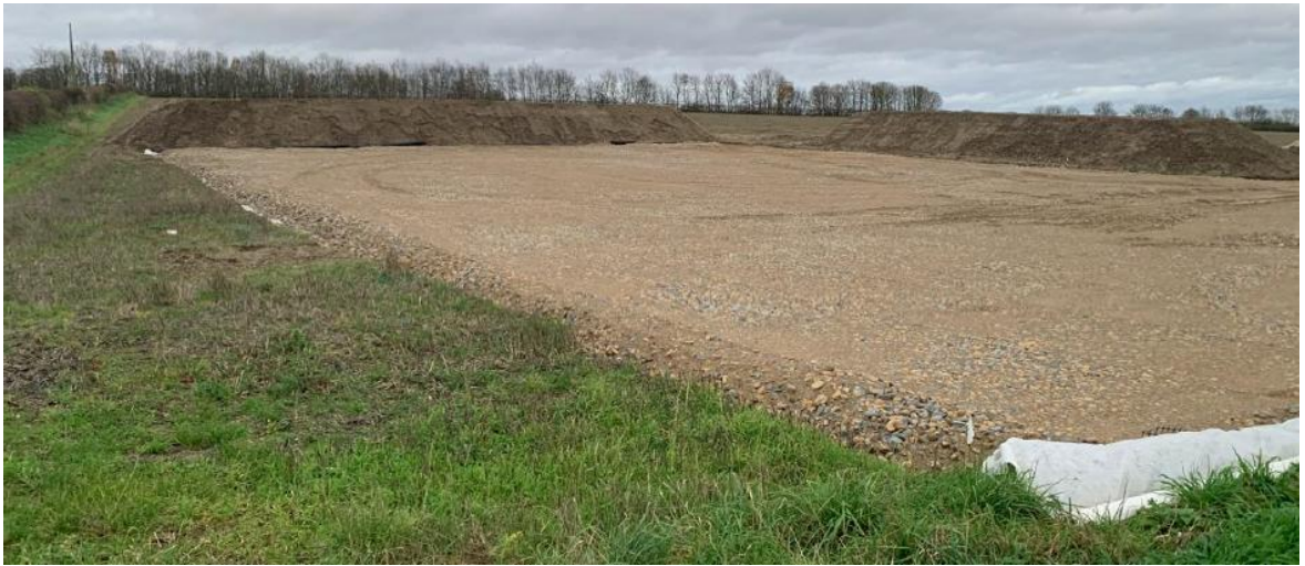
Plate 11-25 Example Construction Compound (being built)
