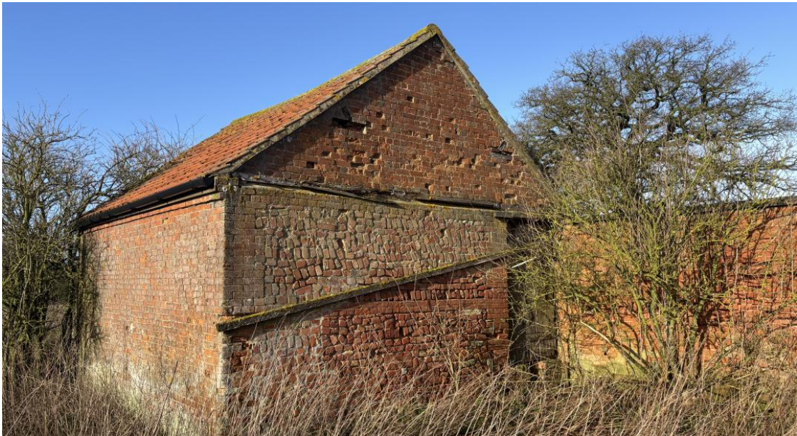
Plate 11-22 Brick Building Within the Site (Field 3)
