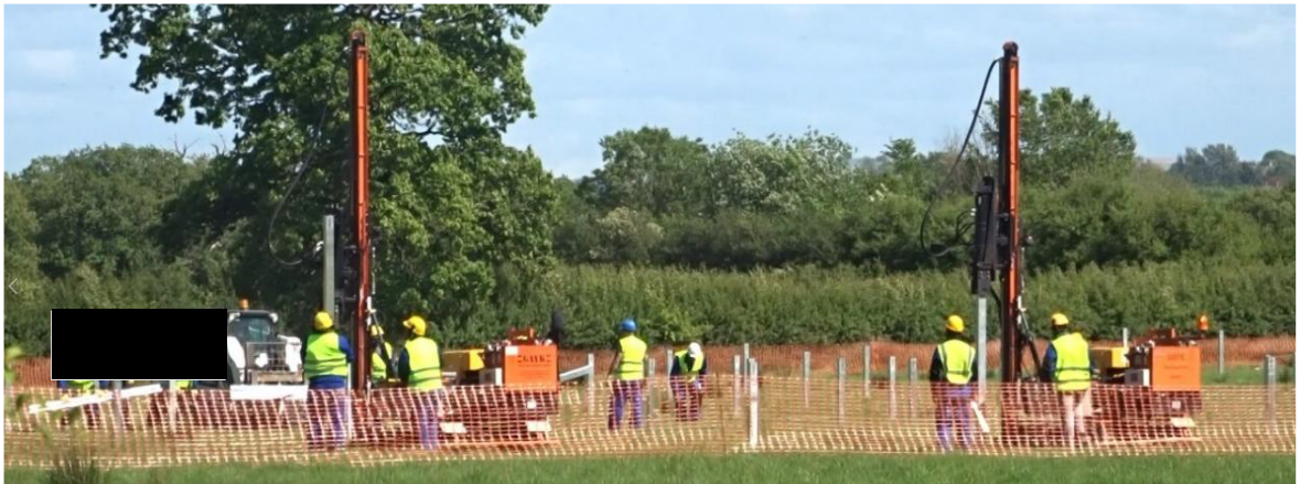
Plate 11-27 Mounting Structure Piles being Installed
