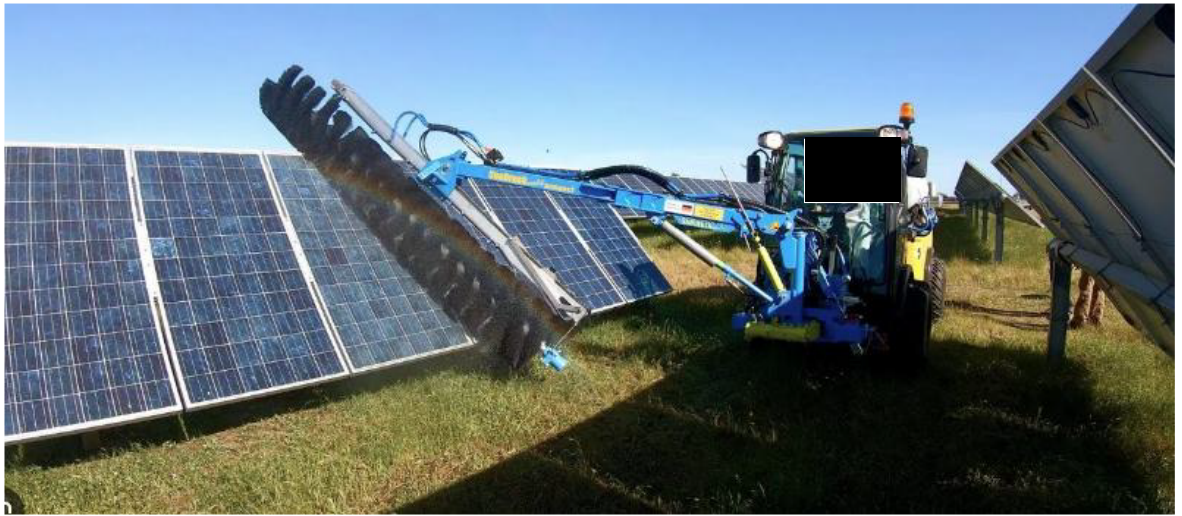
Plate 11-40 Cleaning of Solar Modules
